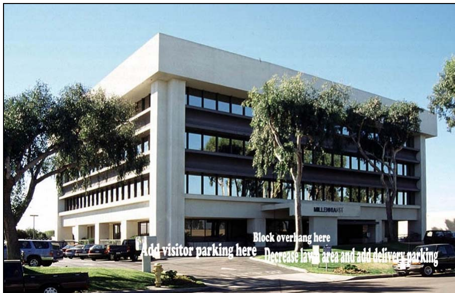
Building “Before” picture with recommendations for parking and circulation
